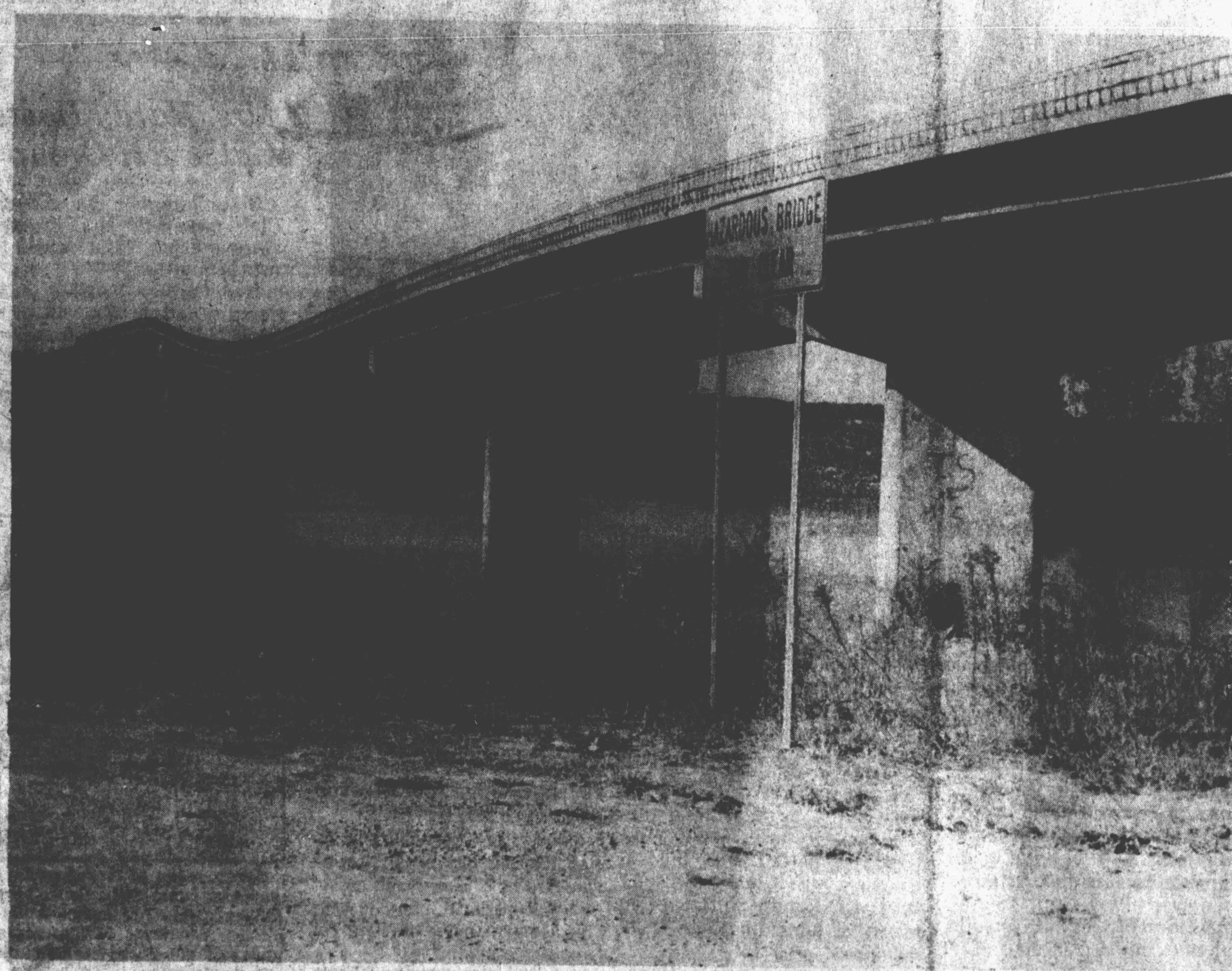
THE CENTER PIER was removed from under the sagging Great River Road Bridge at Hale's Point over the Obion Forked Deer Rivers last week. After an attempt at blasting the support failed, several bulldozers pulled the pier down.
